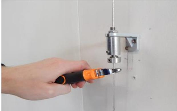
10. Cut out the excess of the cable.
