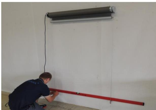
11. With a spirit level mark the installation place of the second cable guide bracket. Other actions make analogically to the first bracket and guide.
