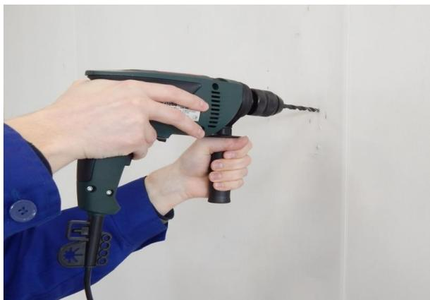
2. Drill holes for chosen fixing system.
