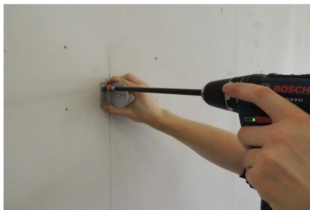
4. Mark places for holes and install second bracket to the wall/ceiling.
