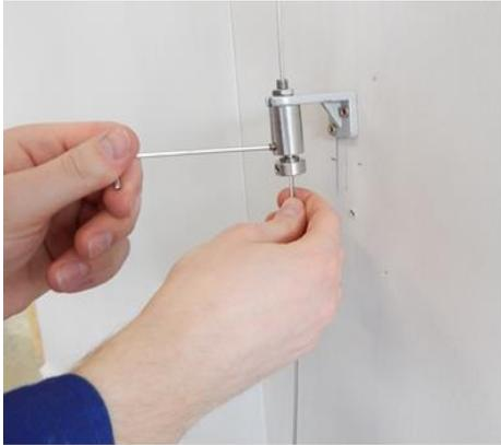
8. Loosen upper screw (locking movable part of the tightener).
