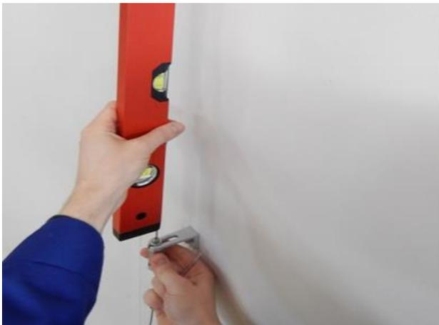
9. Check the vertical level of the cable. If necessary, correct by moving tightener in the bracket.
