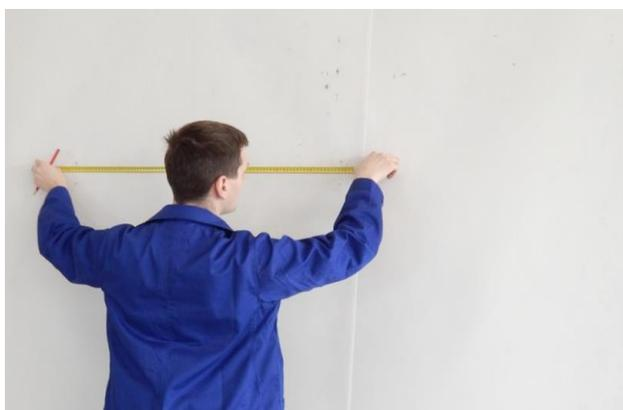
1. Measure and mark installation places for wall-ceiling brackets.
