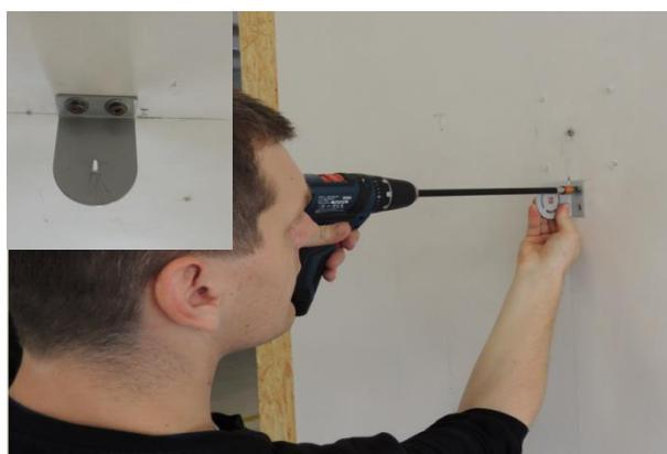
3. Install first bracket to the wall/ceiling, adjust if necessary.
